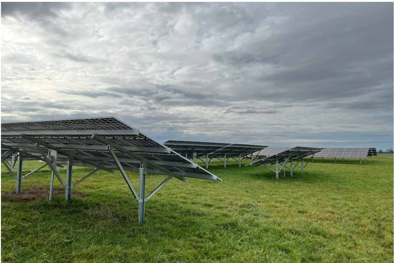
Solar panels have been installed facing three directions to maximise production throughout the day. (ABC Rural: Peter Somerville)
