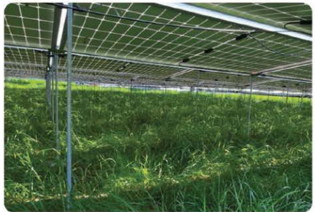
Vegetation (ryegrass) growing beneath a PEG array at the Junee Solar Farm
